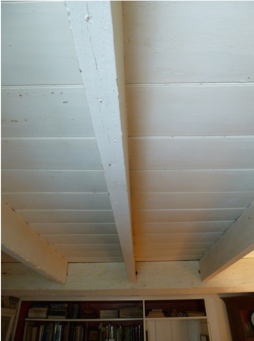
43. Long room ceiling joists, which are smooth-cut. This was a more expensive way to produce joists (pit sawn), compared to the hand-hewn ceiling joists upstairs.
