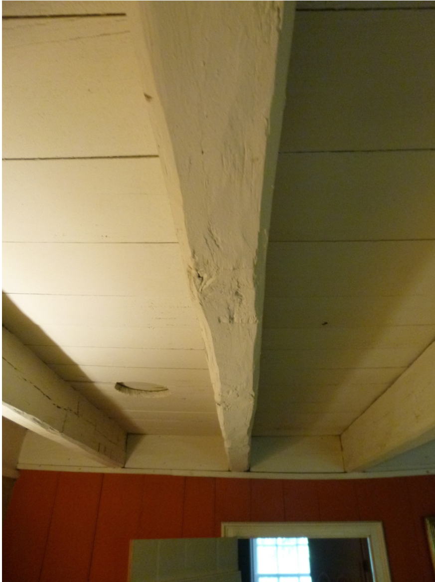
69. Upstairs bedroom ceiling joists, which are hand-hewn. This was a less expensive way to produce joists, compared to the smooth-cut, pit sawn joists downstairs. Door leads to the upstairs bathroom.
