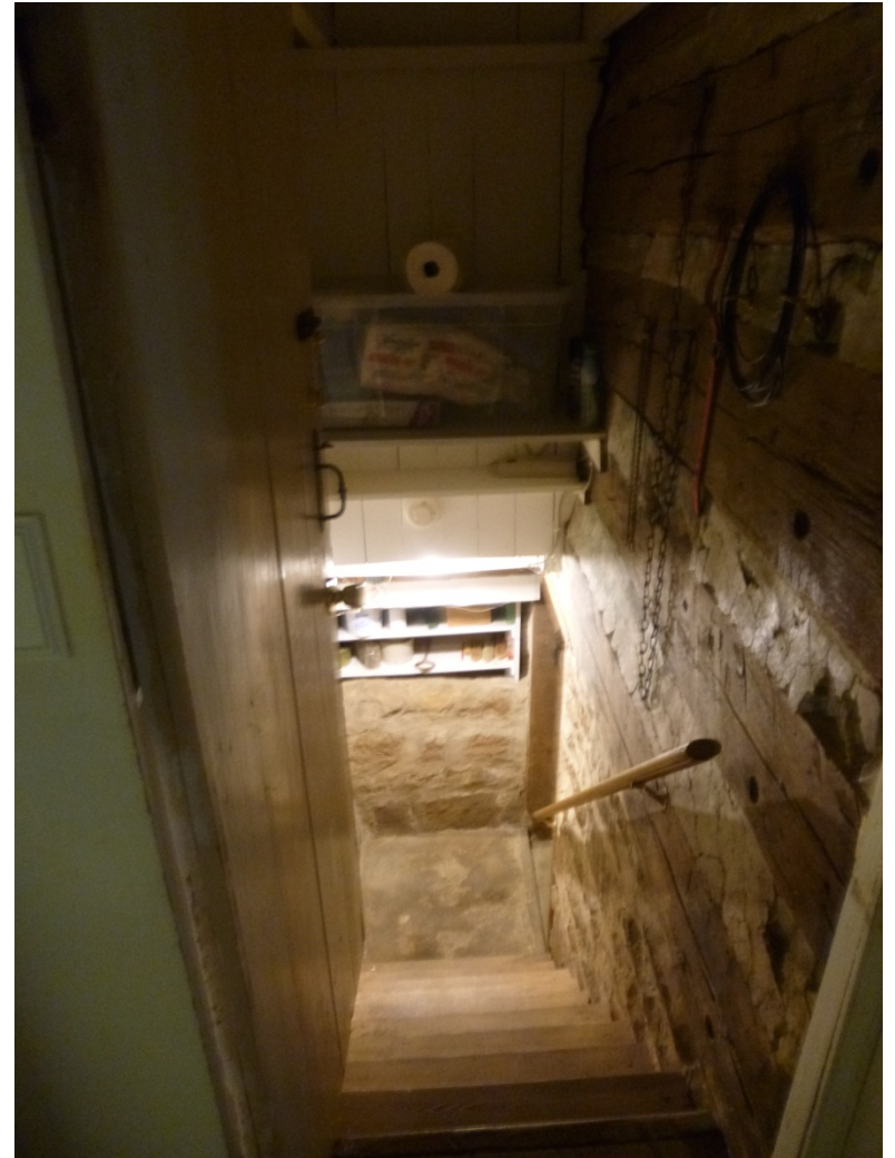
34. Stairs down to the basement. Log wall of original structure visible on wall.
