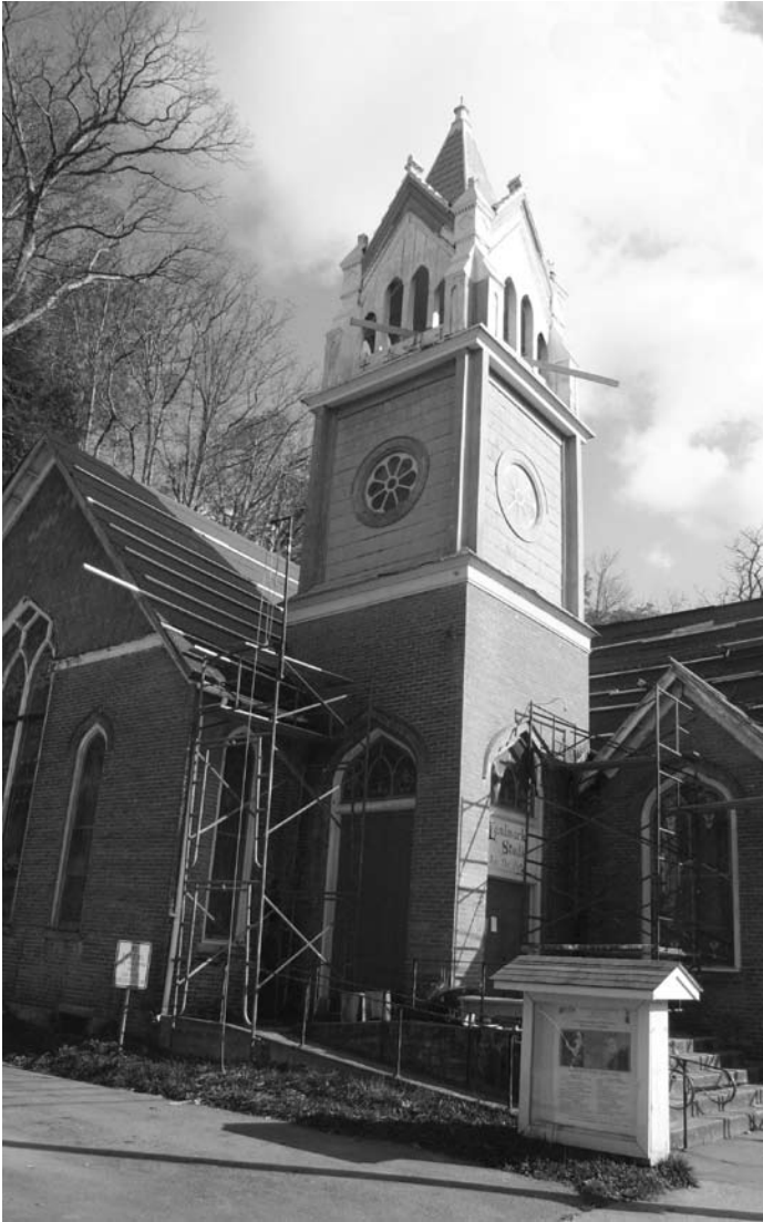
Landmark Studio for the Arts, Sutton photograph by Jeff Pierson
