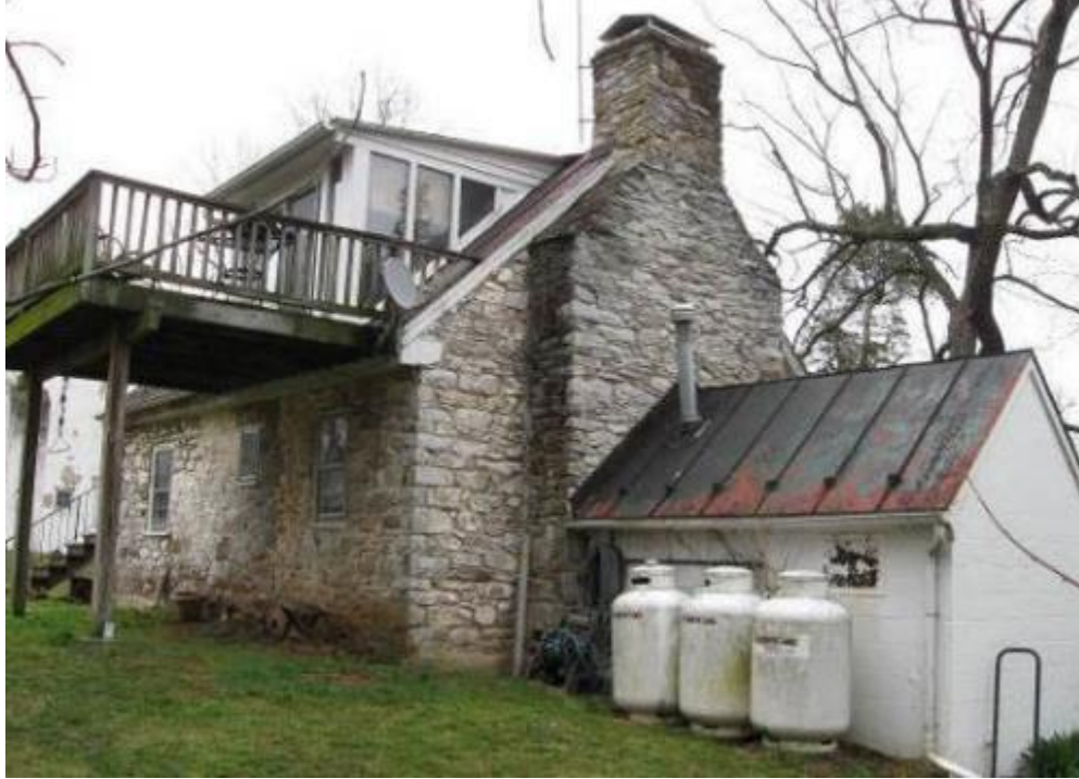
Photo 8: The Rocks, Jefferson County, WV Overseer's House, west elevation, view to southeast showing ell, outboard chimney, second story deck, and shed dormer.
