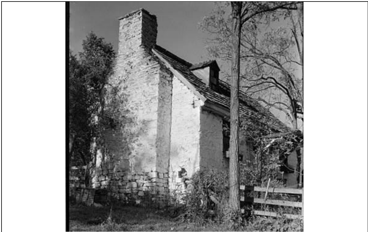
Figure 9. Overseer's House. HABS photograph, 1937, view to northeast.
