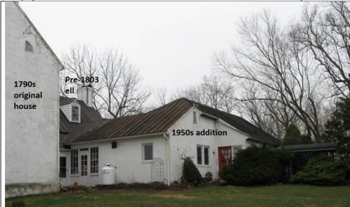
Photo 6: The Rocks, Jefferson County, WV Oblique view to west showing more detail of 1950s addition.
