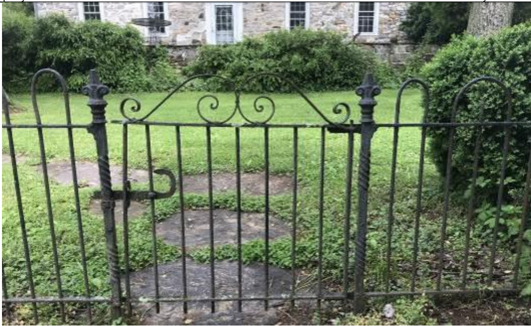
Photo 2: The Rocks, Jefferson County, WV Detail of entry gate and metal fencing. View to northwest
