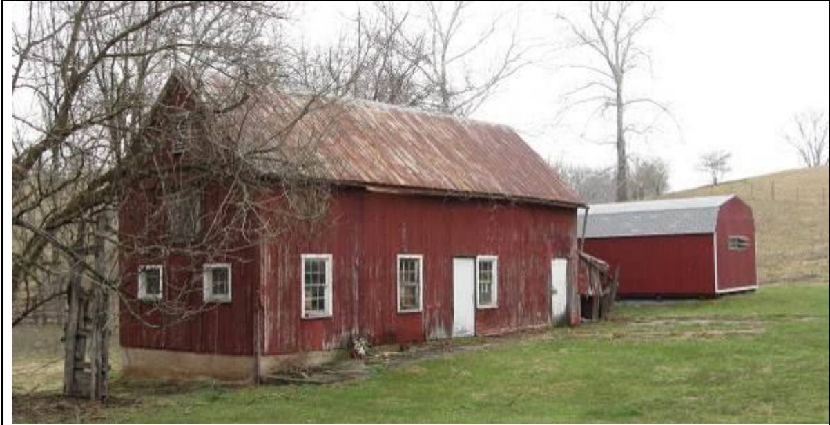
Photo 16: The Rocks, Jefferson County, WV View to northwest of goat barn and shed with gambrel roof.
