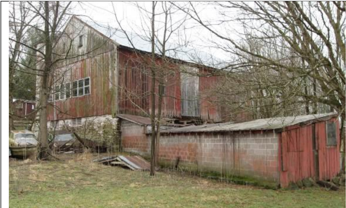
Photo 15: The Rocks, Jefferson County, WV Bank barn, view to southwest showing west gable and cinderblock backside of stables ell.
