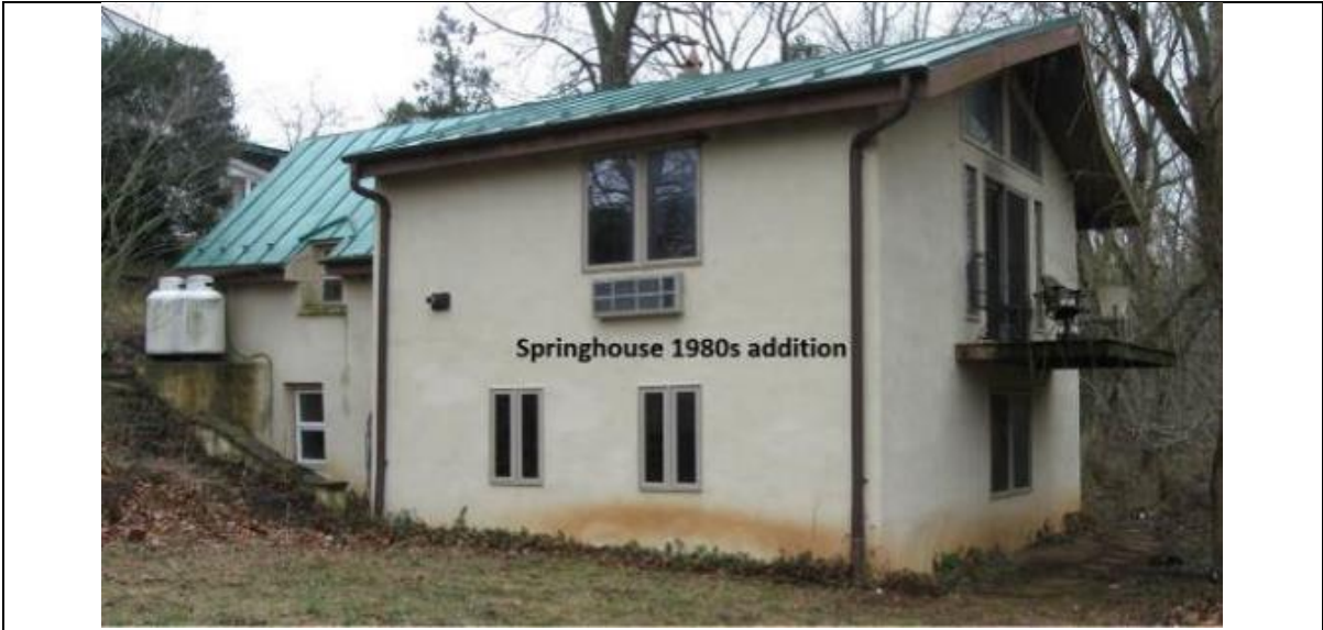
Photo 12: The Rocks, Jefferson County, WV Springhouse, view to southwest showing 1980s addition and second-story cantilevered deck.
