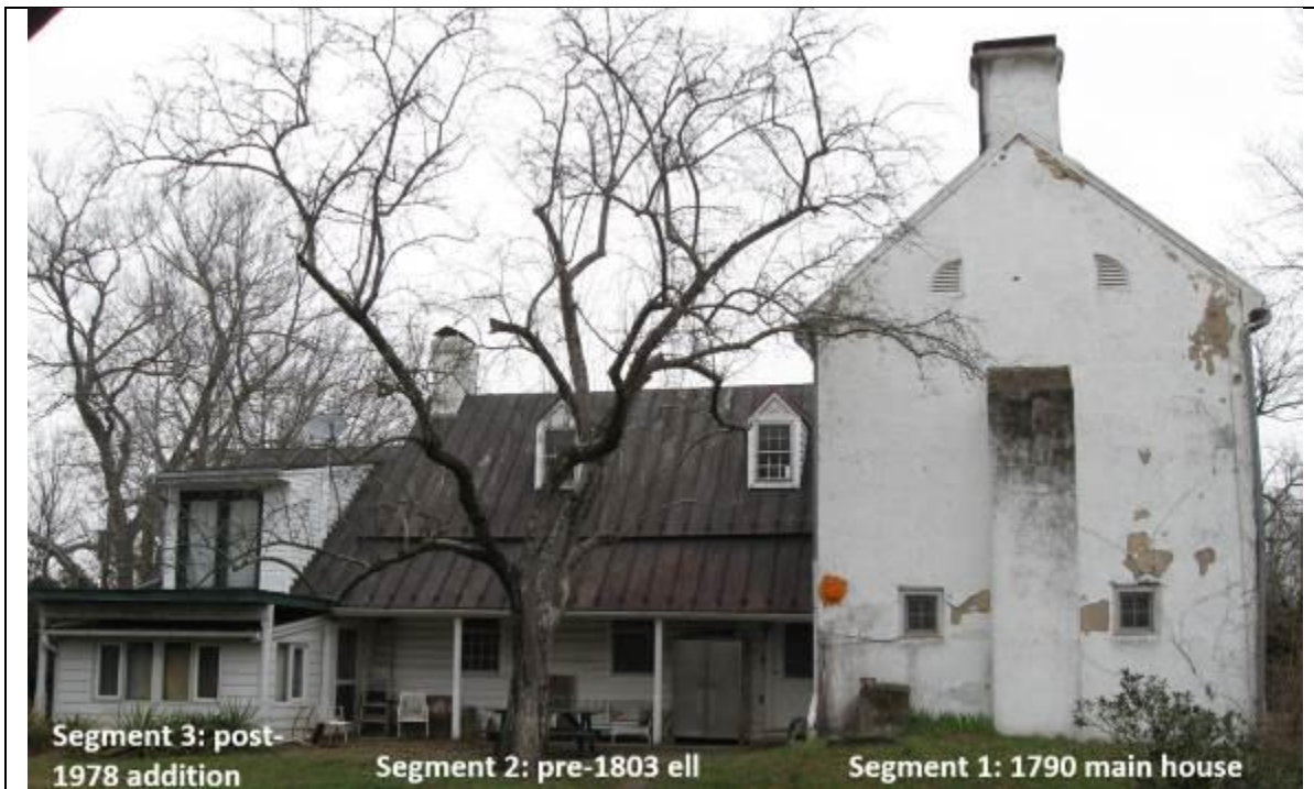
Photo 3: The Rocks, Jefferson County, WV Western elevation. View to southeast of 1790 house, pre-1803 ell, and post-1978 addition.
