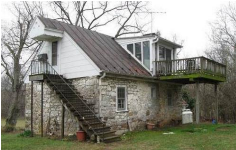
Photo 9: The Rocks, Jefferson County, WV Overseer's House, east elevation, view to southwest showing second story deck, stairs to second story, and shed dormer.
