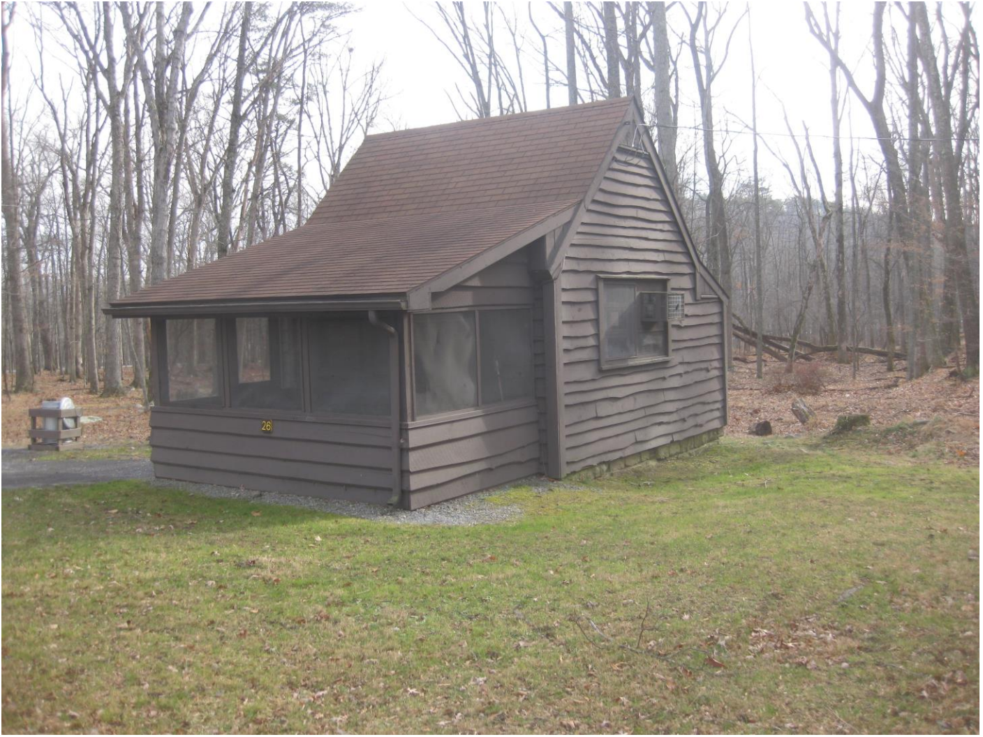
Photo 20: Cabin No. 26 camera facing south
