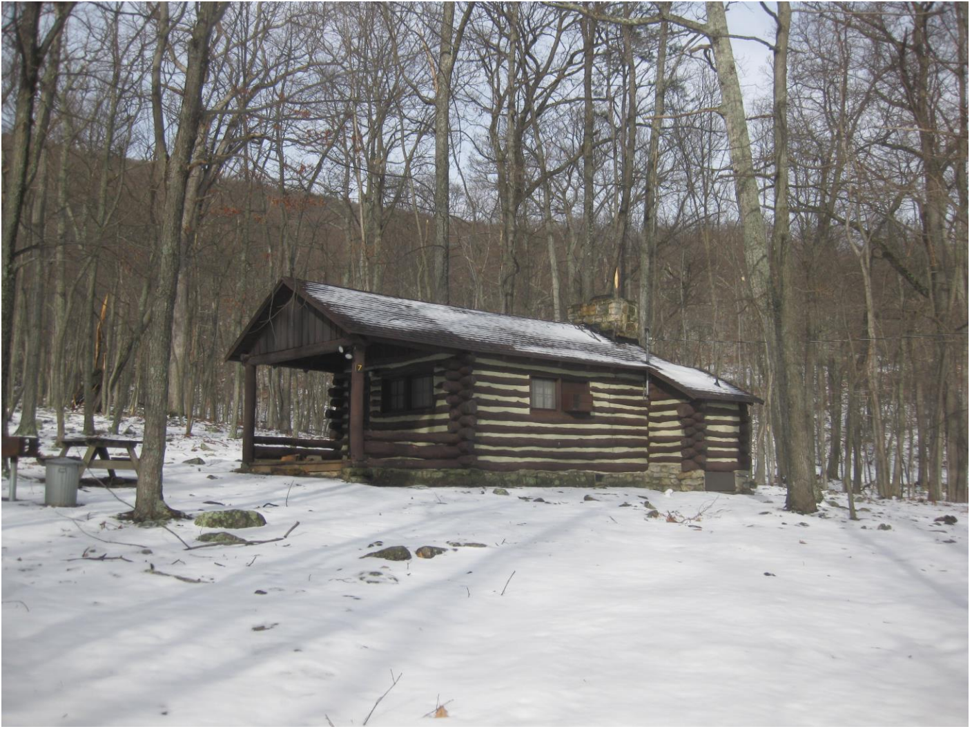
Photo 15: Cabin No. 7, camera facing north
