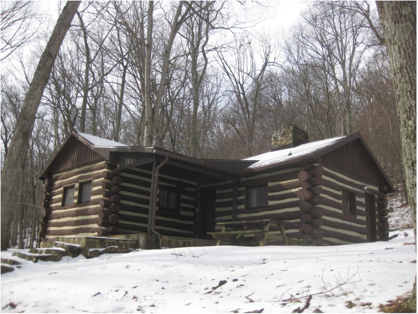
Photo 13: Cabin No. 2, camera facing south
