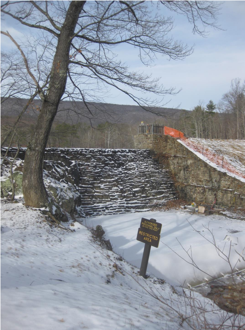
Photo 6: Cacapon Dam, camera facing west
