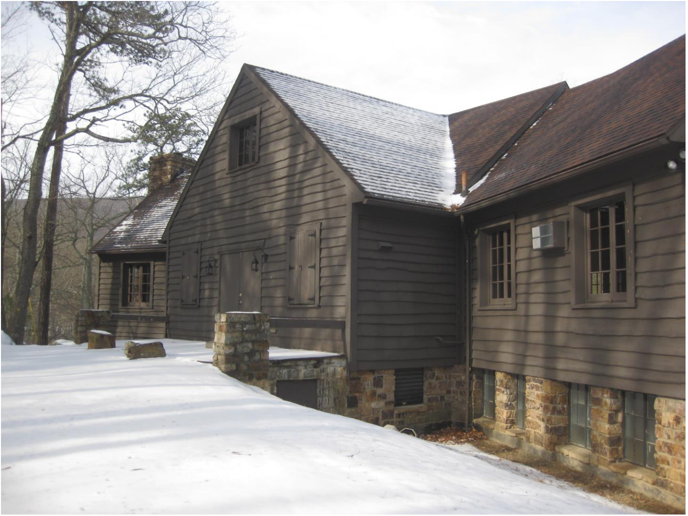
Photo 8: Lake Bathhouse, camera facing northwest
