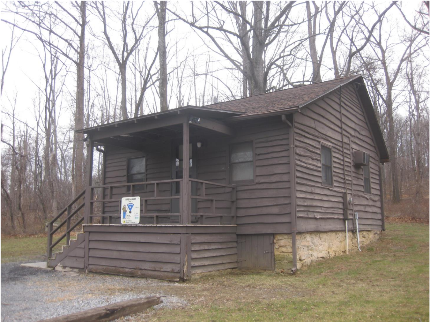
Photo 22: Park Headquarters - Ranger's Residence, camera facing east
