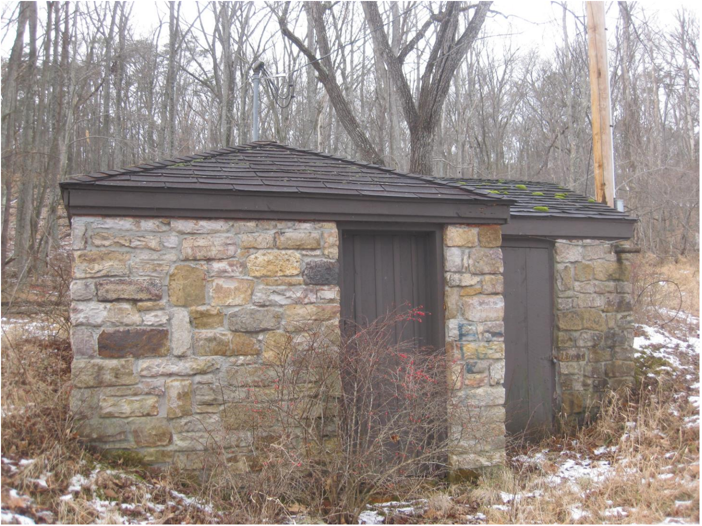
Photo 10: Springhouse, camera facing north
