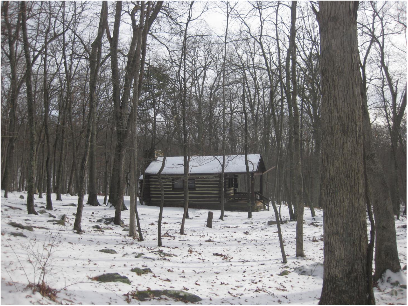
Photo 14: Cabin No. 5, camera facing south
