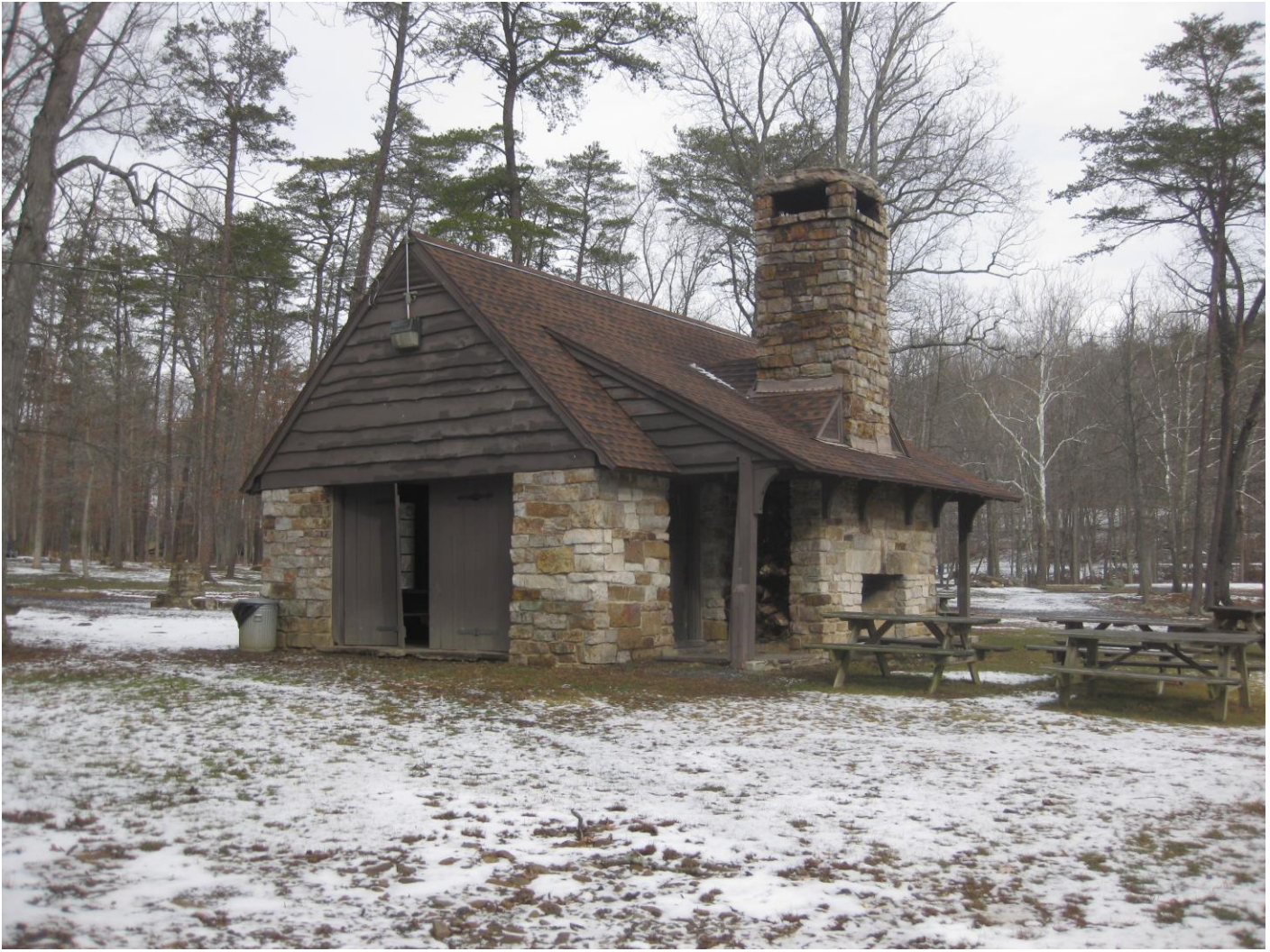
Photo 7: Lake Picnic Shelter, camera facing northeast
