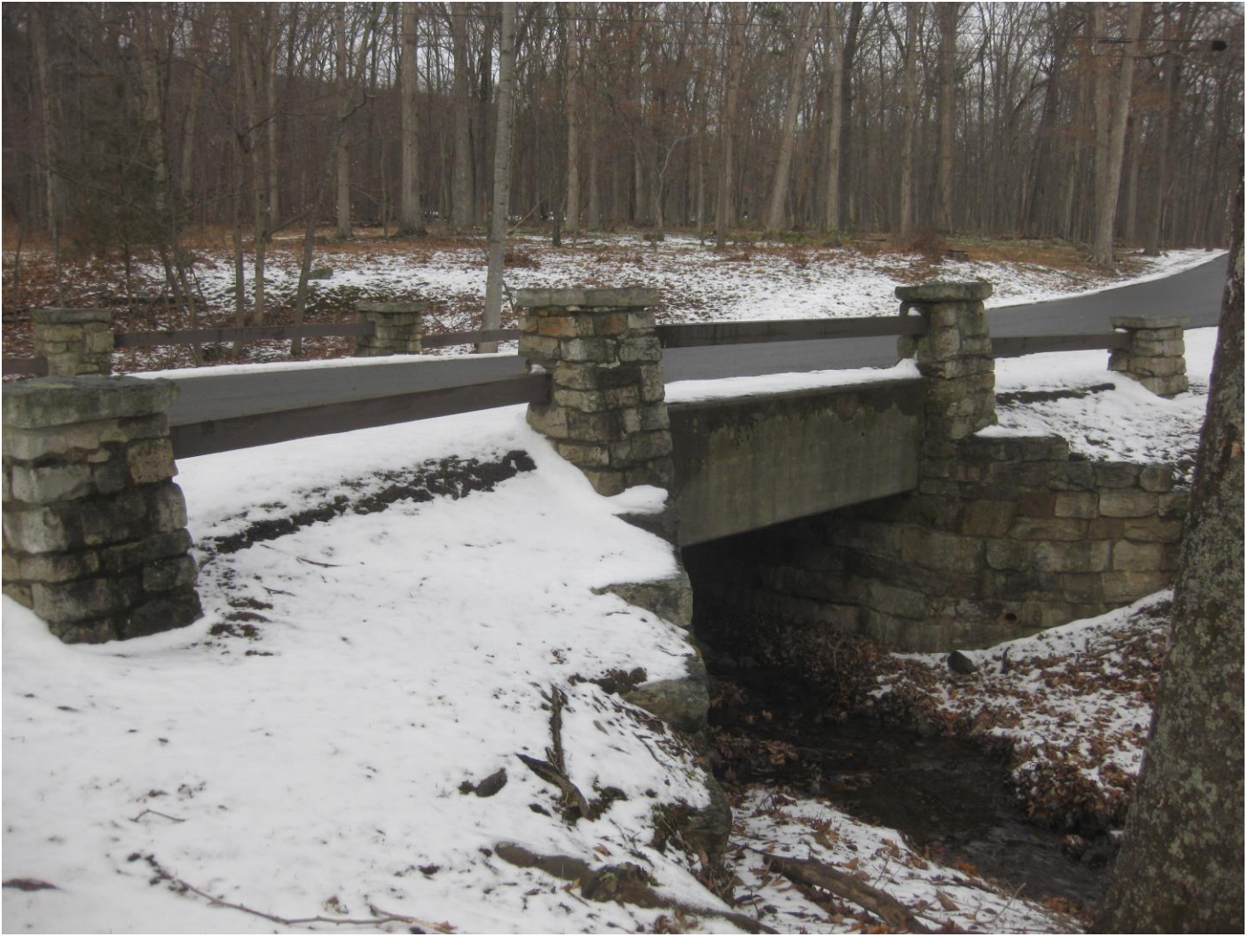
Photo 3: Vehicular Bridge, detail
