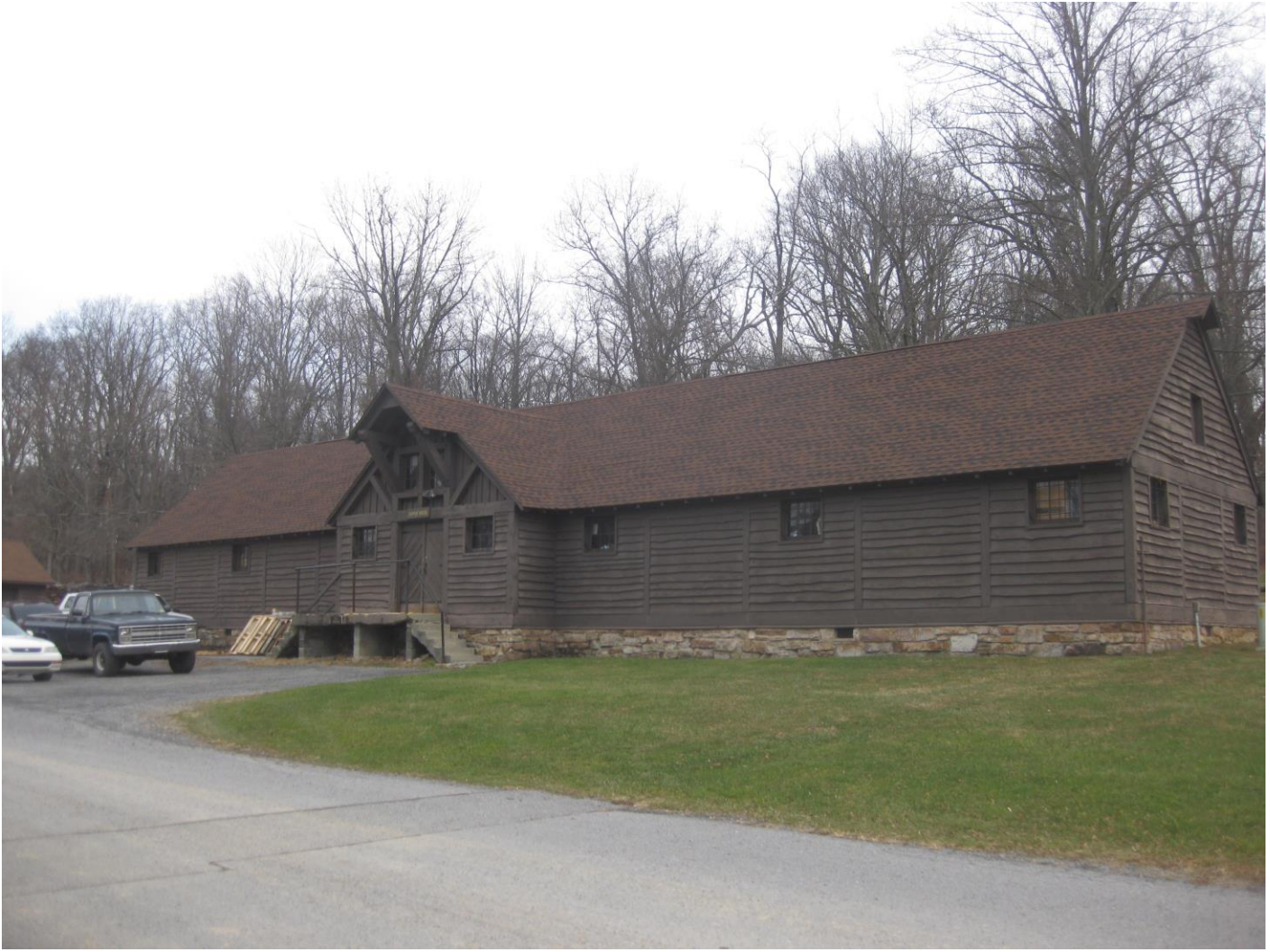
Photo 25: Main Supply House, camera facing northeast
