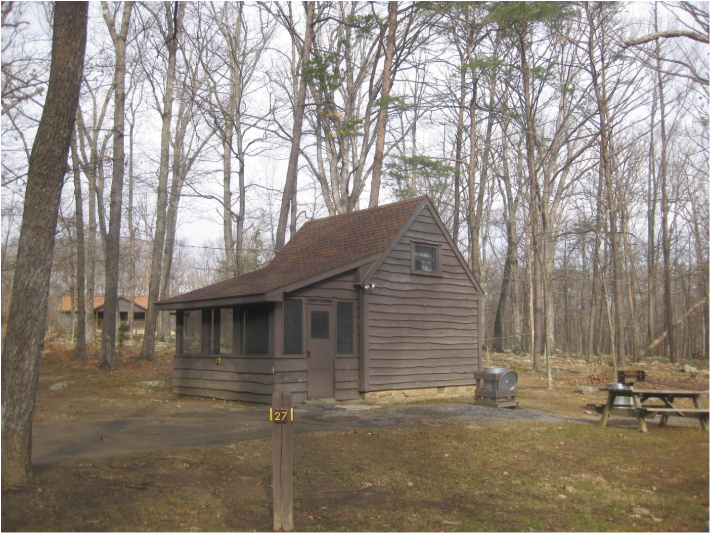
Photo 21: Cabin No. 27, camera facing west
