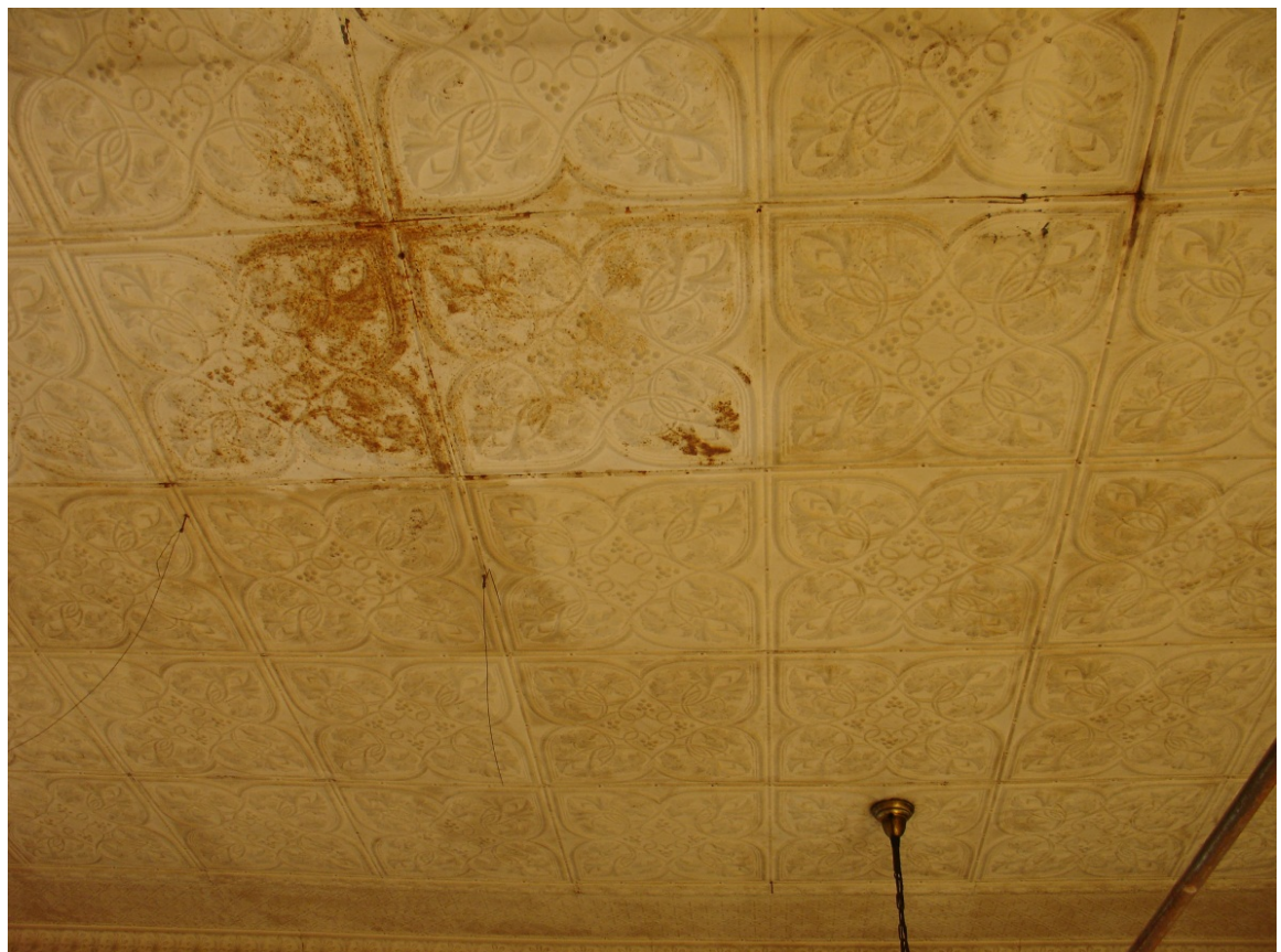
Photo 10: Third floor ceiling
