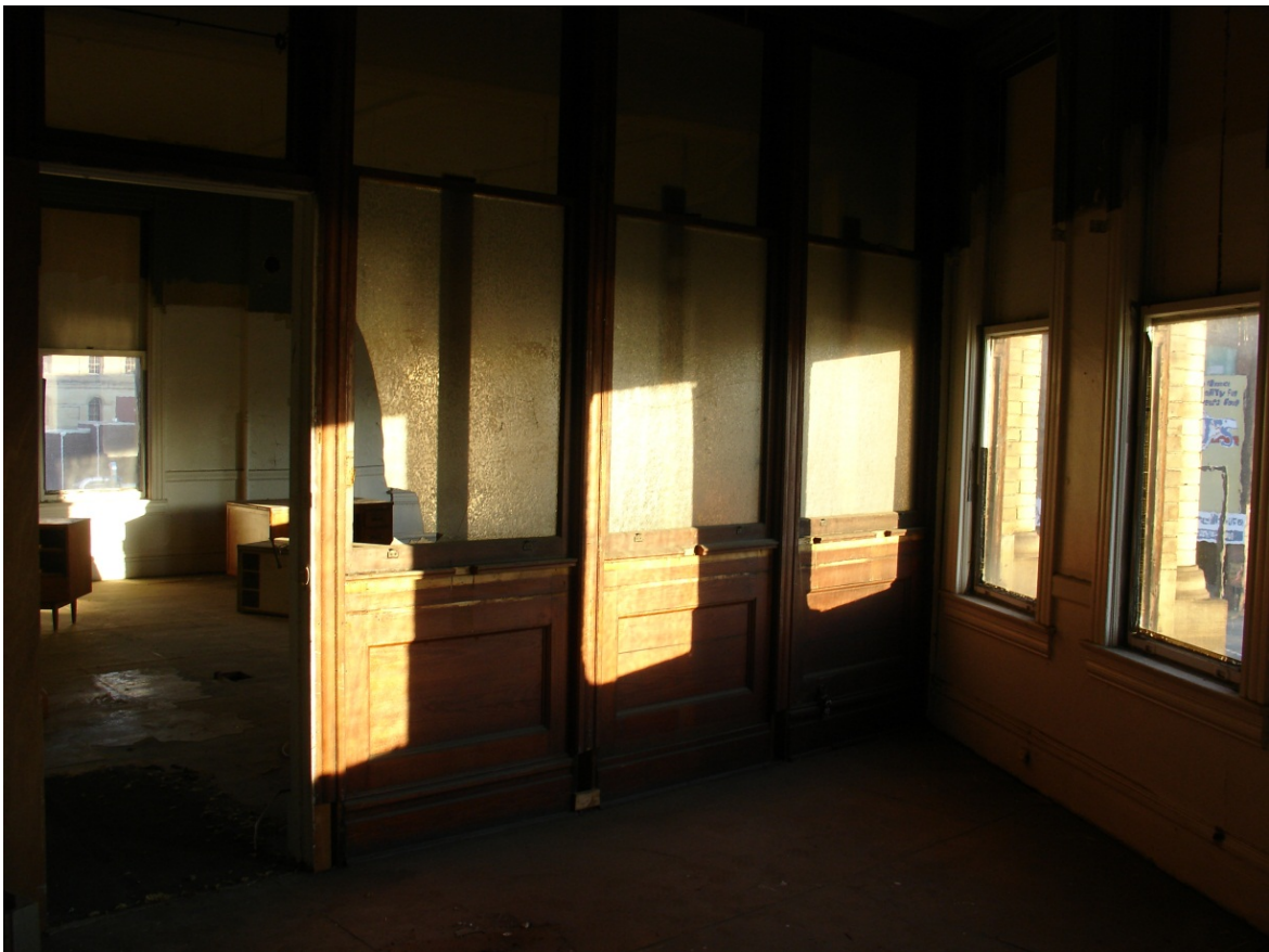
Photo 14: Fourth floor, interior room partition
