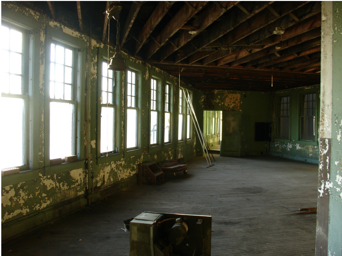
Photo 15: Fifth floor interior (c.1907 addition)
