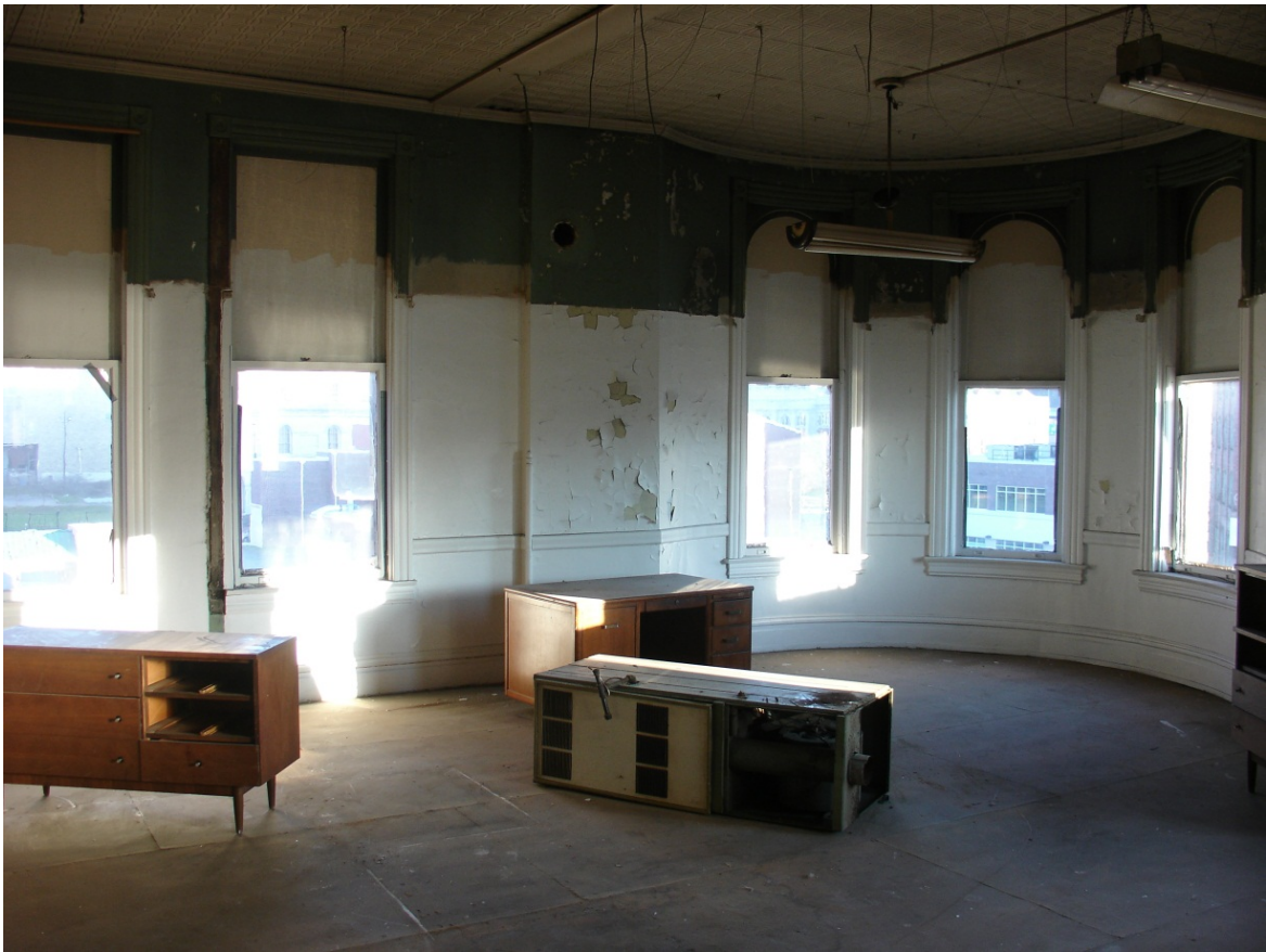
Photo 13: Fourth floor interior showing rounded building corner
