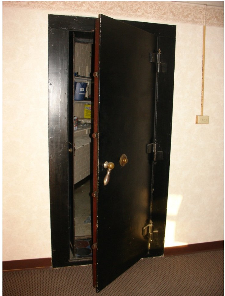
Photo 9: Second floor mezzanine level, vault
