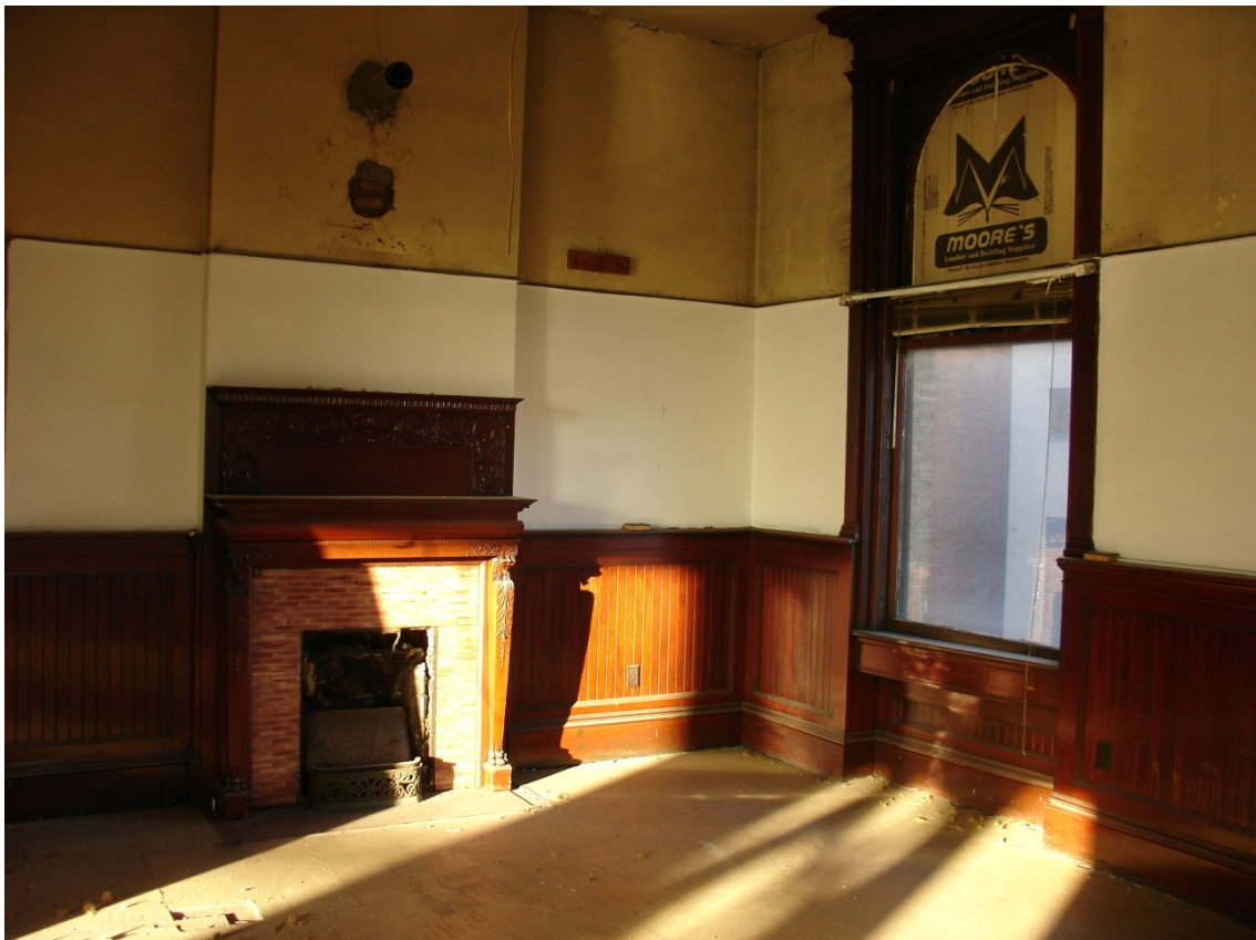
Photo 12: Third floor, gas fireplace and wainscoting detailing
