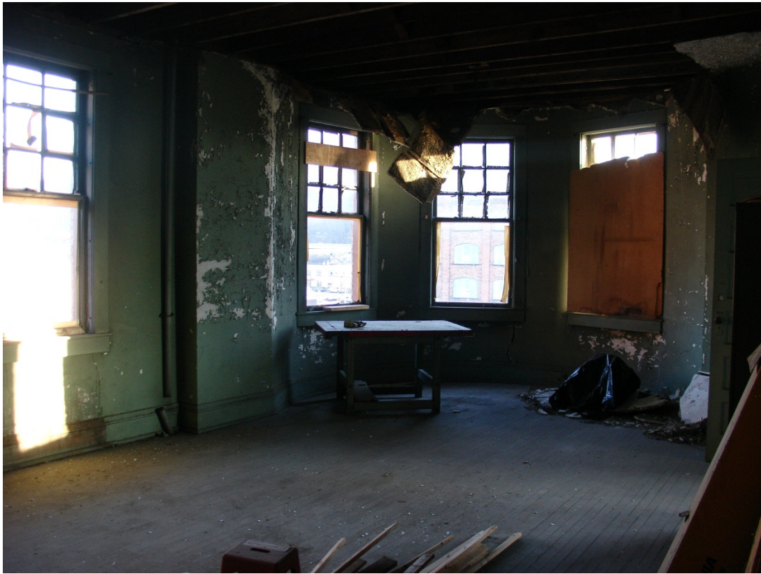
Photo 14: Fifth floor interior (c.1907 addition)
