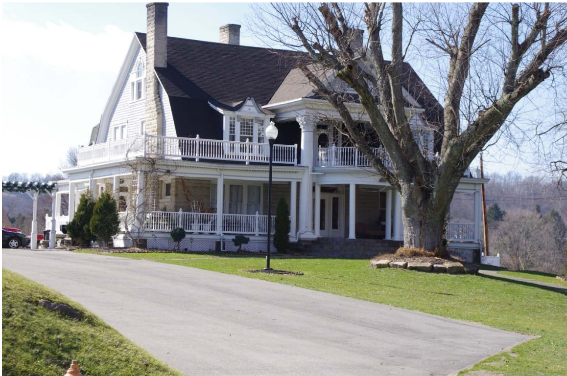
Photo 15 of 26 Resource #175, 75 South Kanawha Street, looking west.
